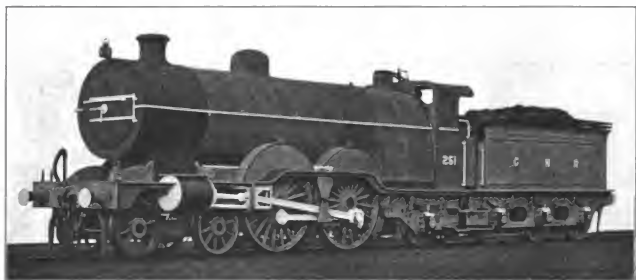
Fig. 5050. Ten-Wheel, Four-Coupled Locomotive. Great Northern Railway. Cylinders 19 in. x 24 in.; Working Steam Pressure 175 lbs. per sq. in.; Total Heating Surface 2,500 sq. ft.; Diameter of Drivers 80 in.; Weight on Drivers 84,640 lbs.; Total Weight 146,720 lbs.
